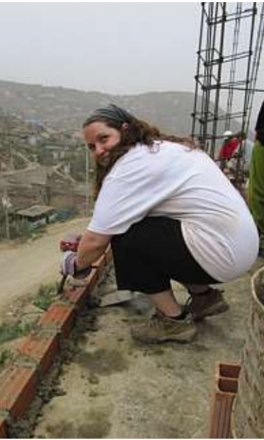
Jen laying brick in Villa Maria de Triunfo.
